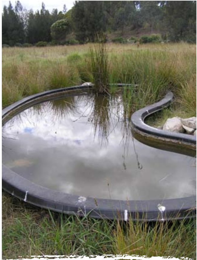
Figure 18: Raised pond with out-turning lip at Sydney Olympic Park
